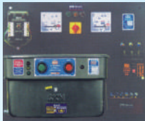
FAB (TPP) CONTROL PANEL
