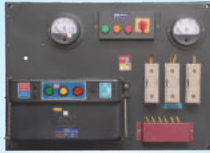
BSA (TPP) CONTROL PANEL
